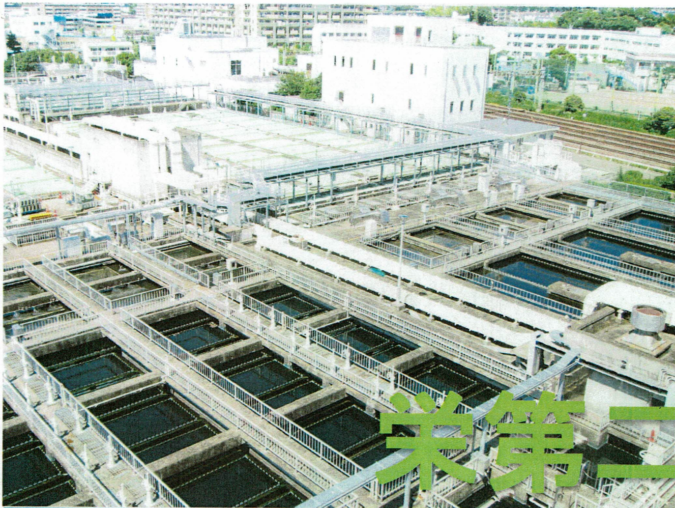
SAKAE II Water Treatment Center
